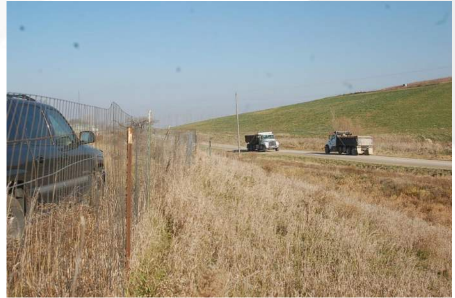
Photo 28 - Phase 2 East Exterior Slope
