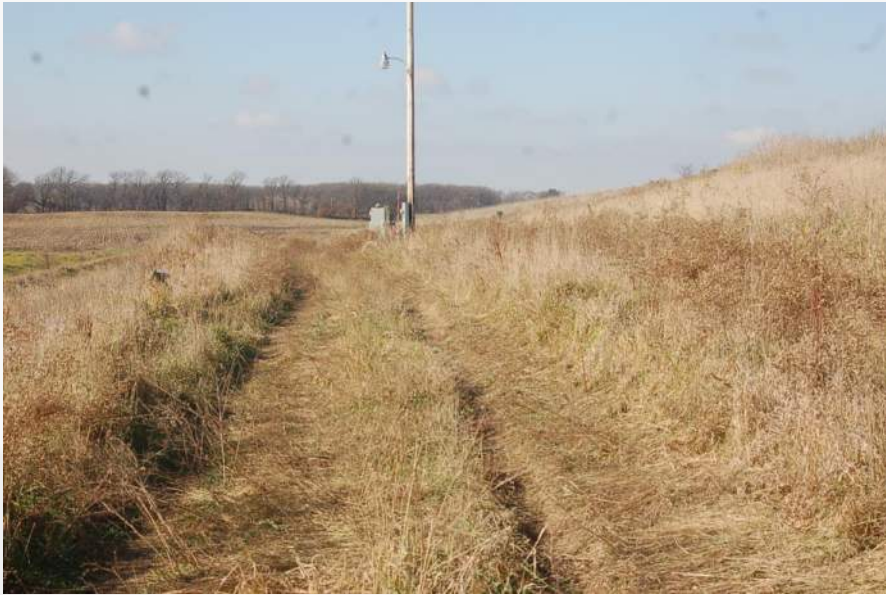
Photo 15 - Phase 2 Top South Berm
