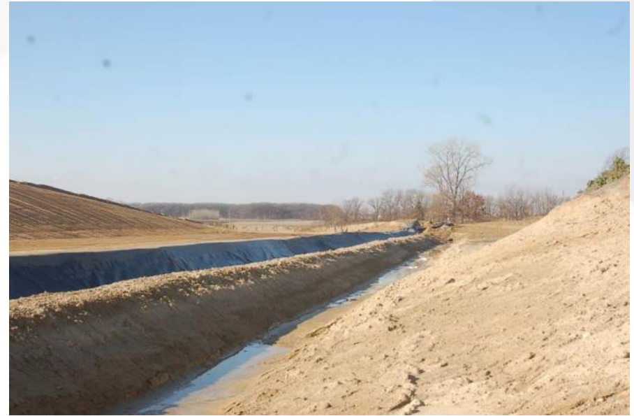
Photo 2 - Phase 3 North Temp Berm
