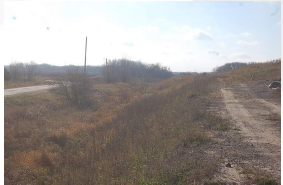
Photo 38 - Phase 2 East Exterior Slope
