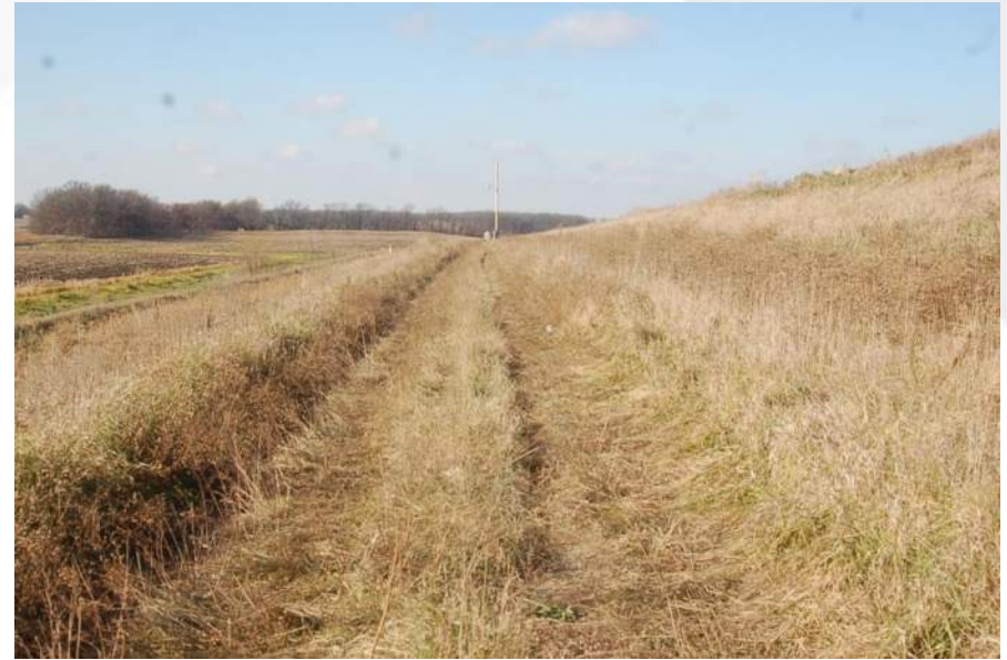
Photo 20 - Phase 2 Top South Berm
