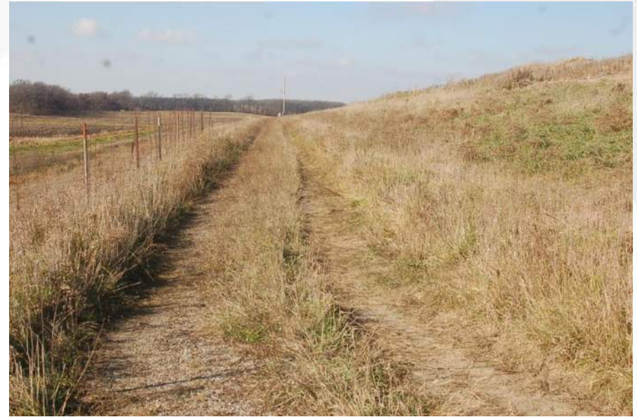
Photo 26 - Phase 2 Top South Berm
