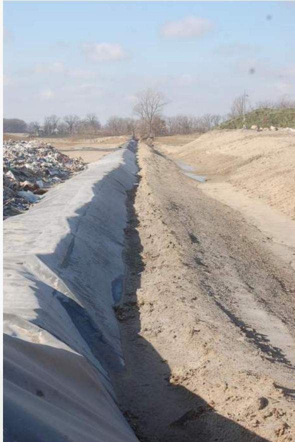
Photo 39 - Phase 3 North Temp Berm
