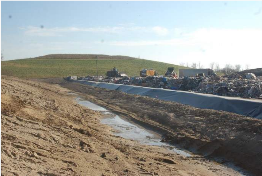
Photo 1 - Phase 3 North Temp Berm
